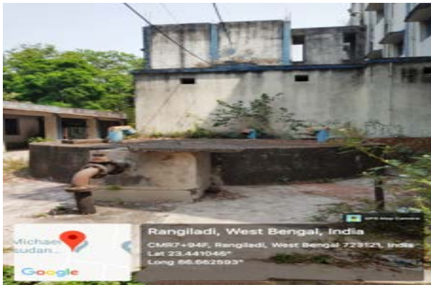
Distribution from 2 nd Reservoir
