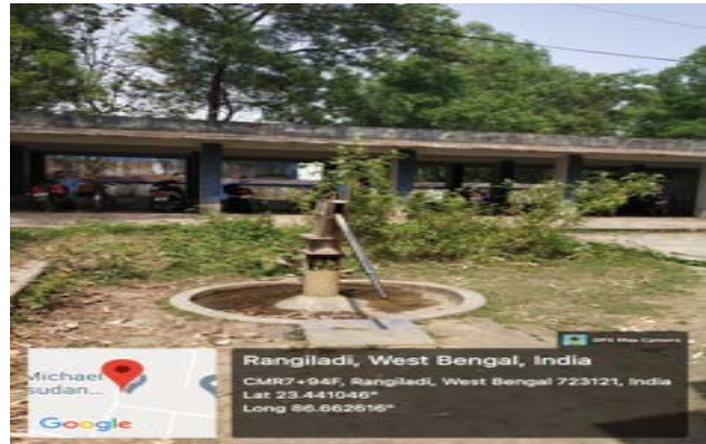
Bore Well (for Drinking)
